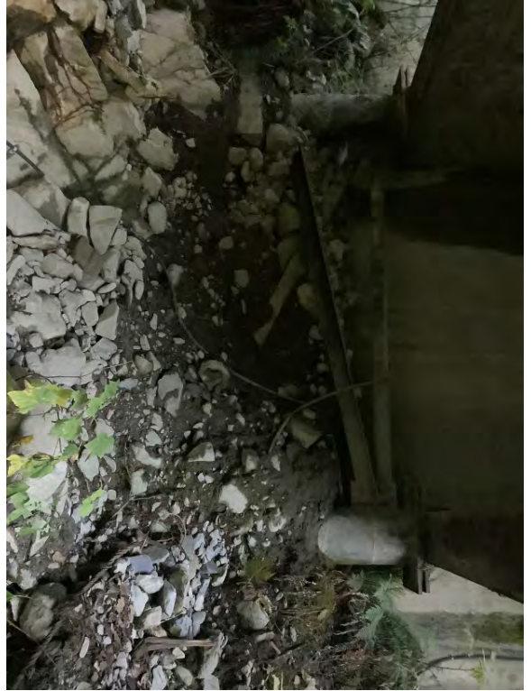
Left Bank Abutment when facing downstream
